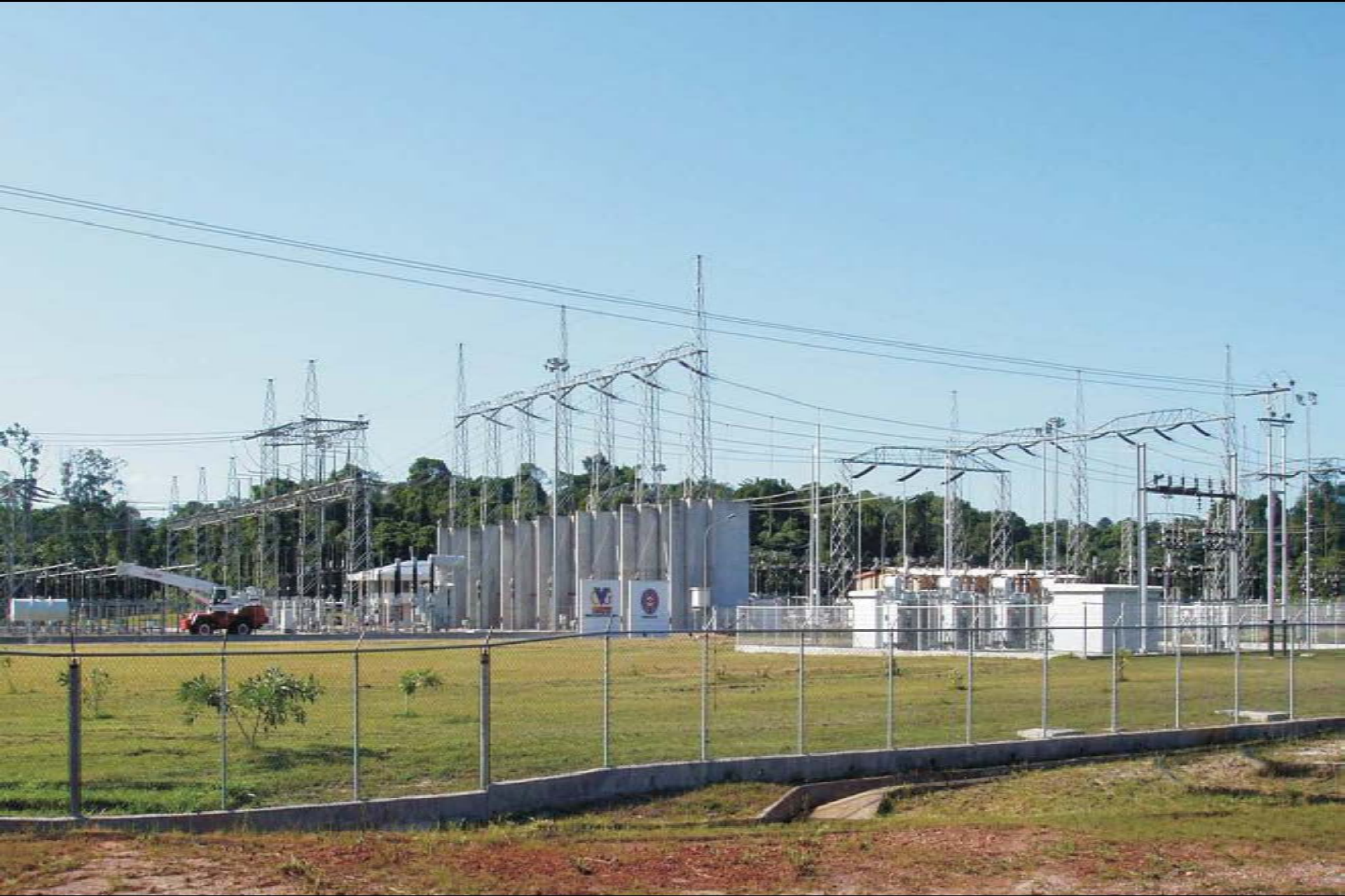
Figure12- The electrical substation that will serve the Las Brisas project.
